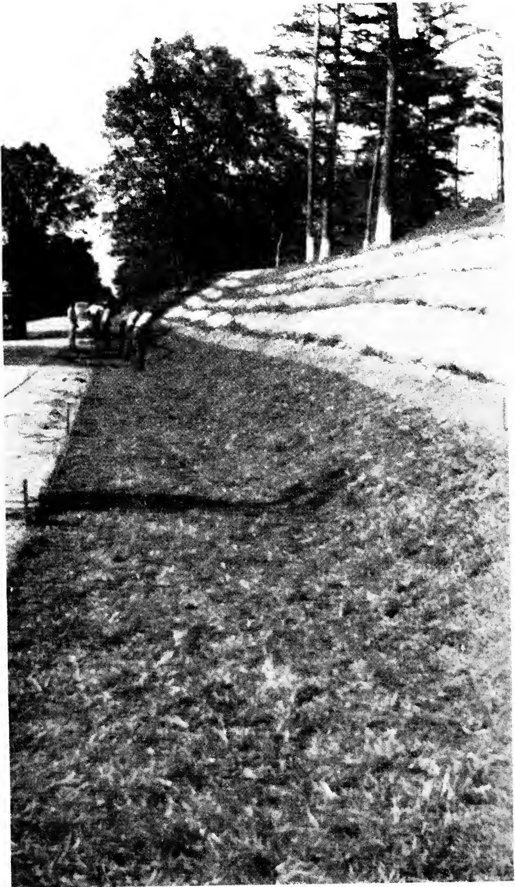
TO CONTROL EROSION ON SLOPES, HONEYSUCKLE IS PLANTED IN CONTOUR TRENCHES. IN GUTTER AREA AND PART WAY UP THE SLOPE SOD IS PLACED. THIS COMBINATION IS EFFECTIVE AS WELL AS ATTRACTIVE
